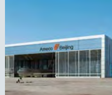
Ameco A380 Hangar Peking, China
