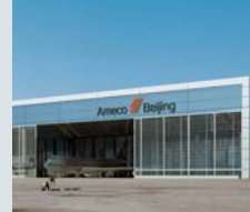
Ameco A380 Hangar Peking, China
