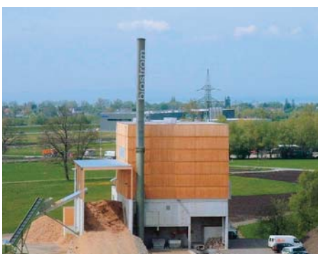
Biostrom Fussach, Österreich Bio-power plant in Fussach, Austria
