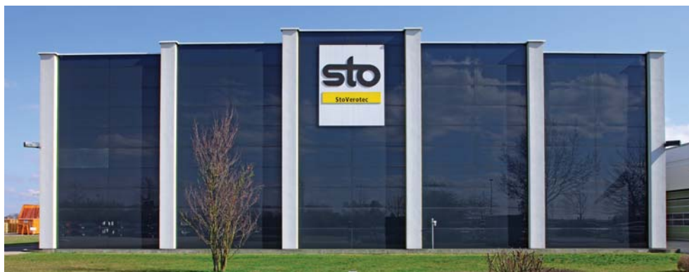
StoVerotec, Lauingen (Donau) StoVerotec, Lauingen (Danube), Germany
